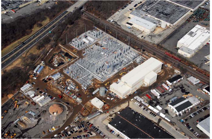
Converter Station at Duffy Avenue, Long Island, Nearing Completion in Spring 2007
